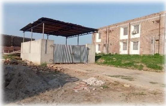
GARBAGE POINT COMPLETED
