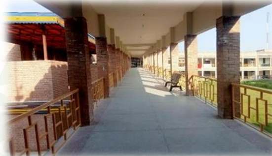
CORRIDOR LINKING WARDS COMPLETED
