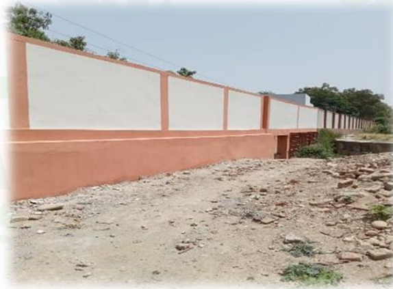
BOUNDARY WALL COMPLETED - THQ TOPI
