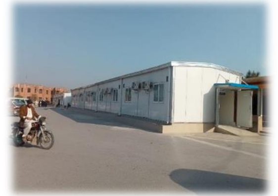
PRE-FAB FILTER CLINICS COMPLETED
