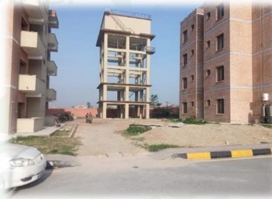
OVERHEAD WATER TANK COMPLETED
