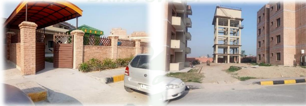
DAY CARE CENTRE COMPLETED
