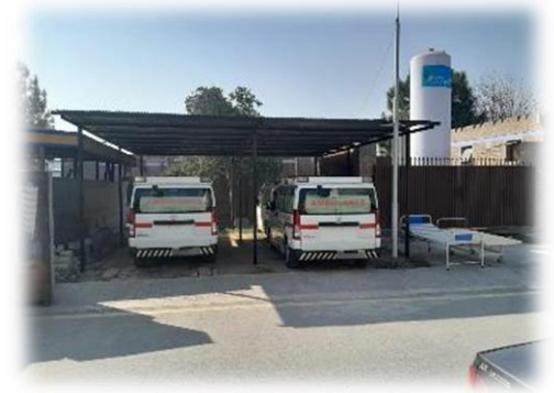
AMBULANCE PARKING SHED
